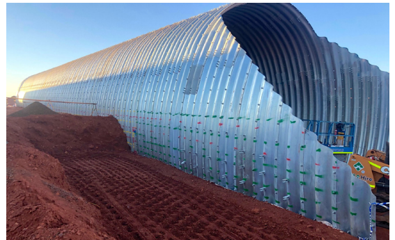
Markings and attachment brackets for soil reinforcement
