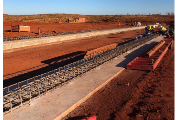
Smaller concrete footings on prepared foundation soils
