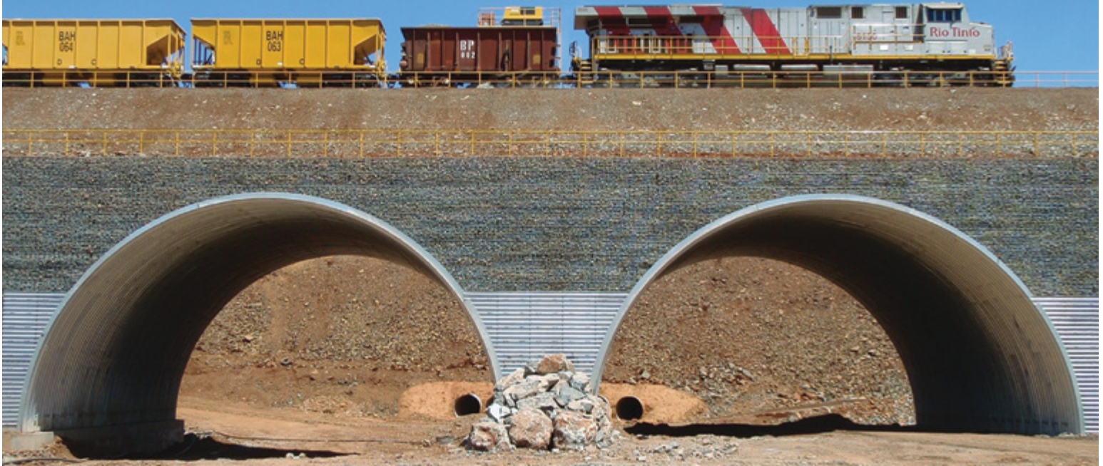
Heavy Haul Rail Crossing, Australia - Super-Cor® Arches
