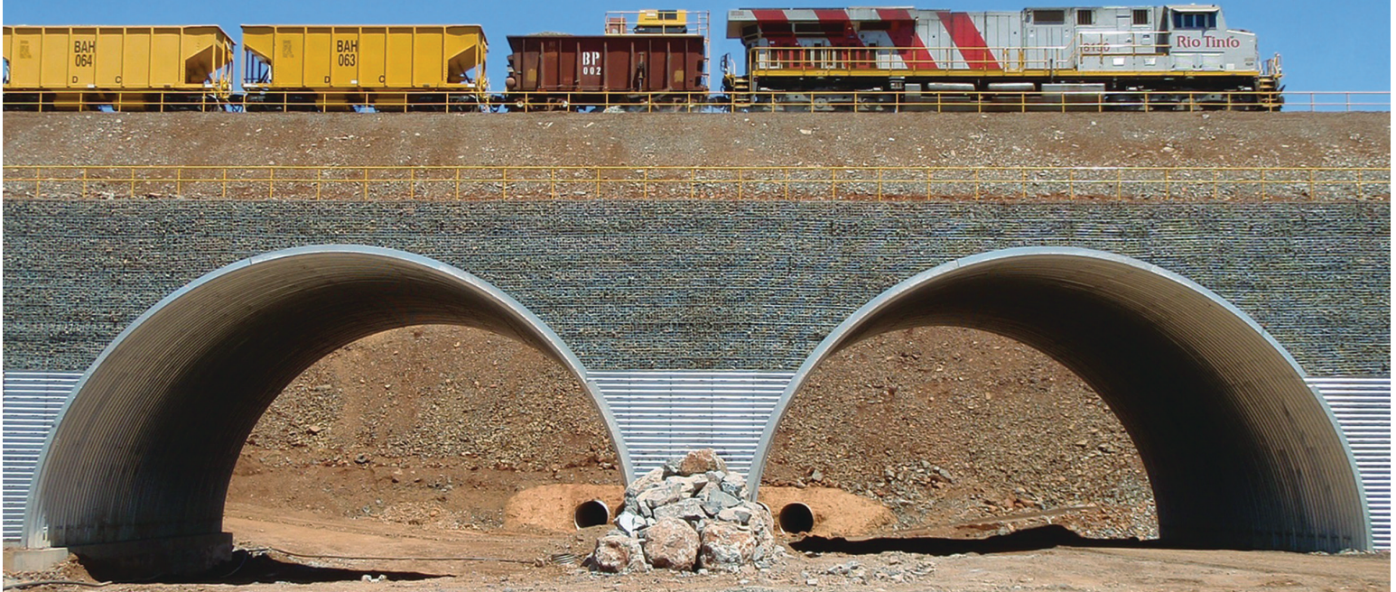
Heavy Haul Rail Crossing, Australia - Super-Cor® Arches
