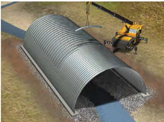
If specified, reinforcement ribs are then added.
