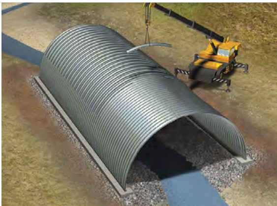
If specified, reinforcement ribs are then added.
