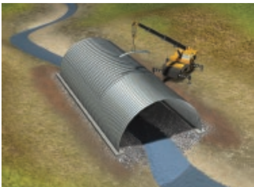
If specified, reinforcement ribs are then added.
