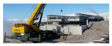
Bolt-A-Bin cells are formed from strong Galvanized and Aluminized Type 2 steel components that are bolted together at the job site and then filled with granular material. The fill material and the metal shell act as a gravity-retaining wall to resist surcharged loading, sliding and overturning of the earth behind the wall.
