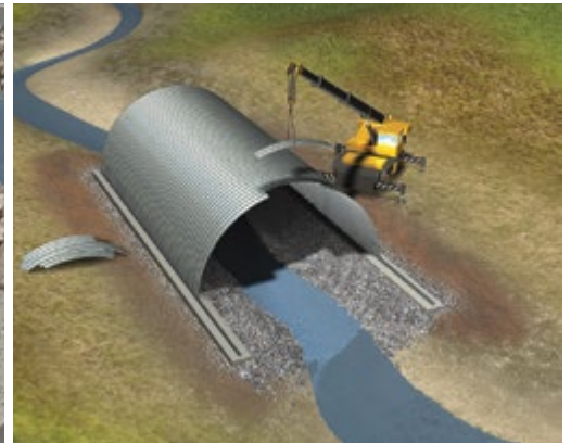
Plates then attach individually to make up other arch segments.
