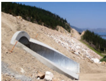
This Bolt-A-Plate® recreational trail and wildlife underpass installed in just eight days. Highway 97, British Columbia.
